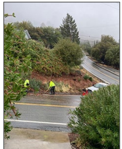
County crew clearing roadside debris in November 2024
